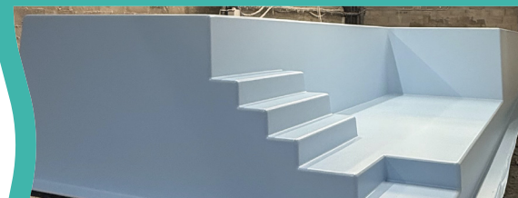
3. Application du barriercoat
